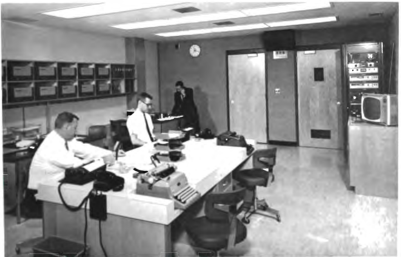
FIG. 22. Nerve center of WOC news room. Microphones on desk provide contact with mobile units. Twelve receivers on wall shelf monitor area emergency frequencies. (Spot news recording is at right. This rack is duplicated in the studio, and tapes in both racks are remotely controlled from the studio console.)
