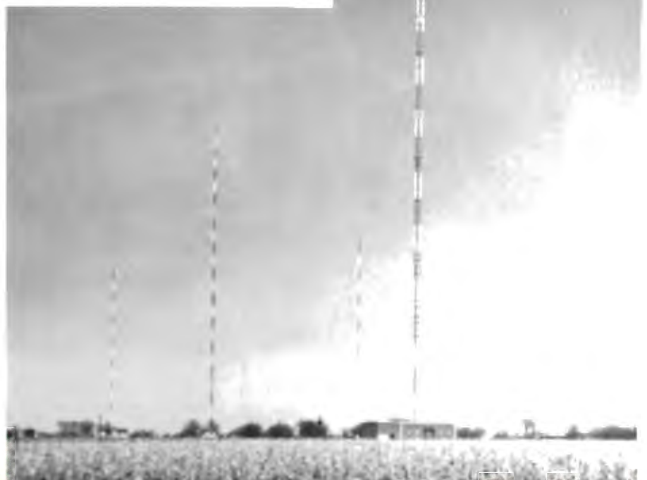
FIG. 38. In 1961 the new transmitter building was completed. New equipment, all RCA, was installed. Foreground tower radiates TV signal. Three tower array in rear radiates AM signal.
