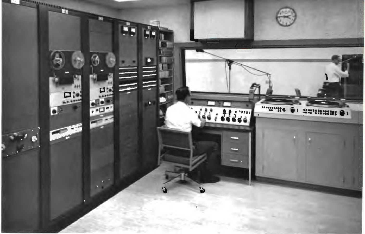
▲ FIG. 34. WOC Radio Master Control. Equipment includes turntables, disc-cutting units, reel-to-reel tape and cartridge tape. Entire radio operation is transistorized.
